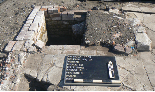
Brick-lined privy inside an outbuilding with a concrete floor at 219 South Miro Street.
