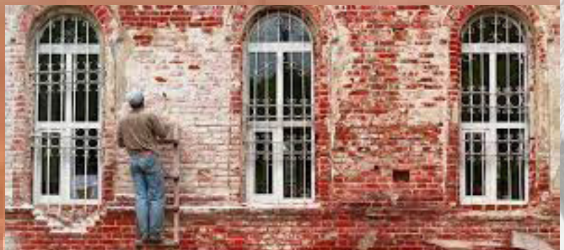
MASONRY REPAIR, REPOINTING, AND CLEANING
