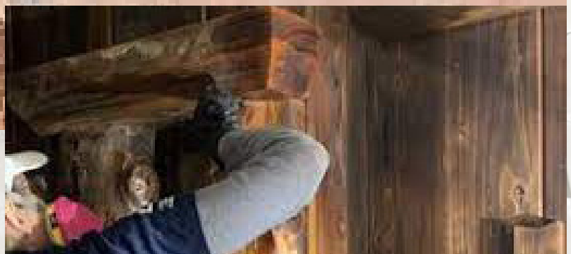
WOOD REPAIR AND REPLACEMENT
