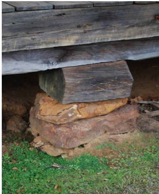
Photo 29. Ironstone and wooden block pier.
