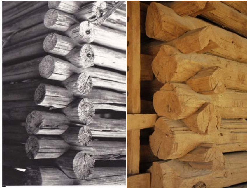
Photos 24 & 25. Saddle notching (left), with a U shape cut. V notch (right).
