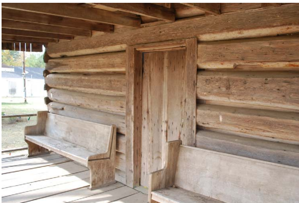
Photo 8. Façade construction detail – Florien single pen log house.
