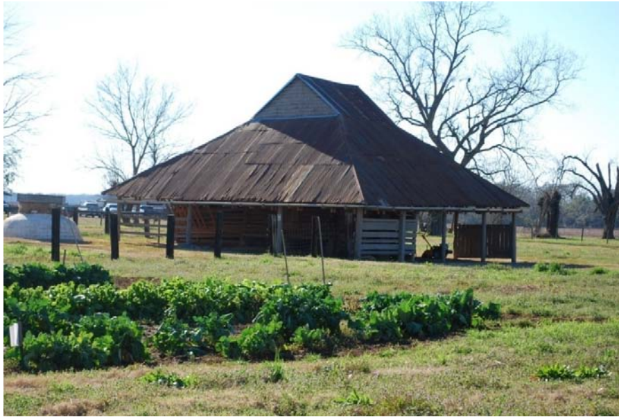
Photo 20. A mid-nineteenth century barn at Oakland Plantation, Natchitoches Parish, with a two story log single crib at the core.
