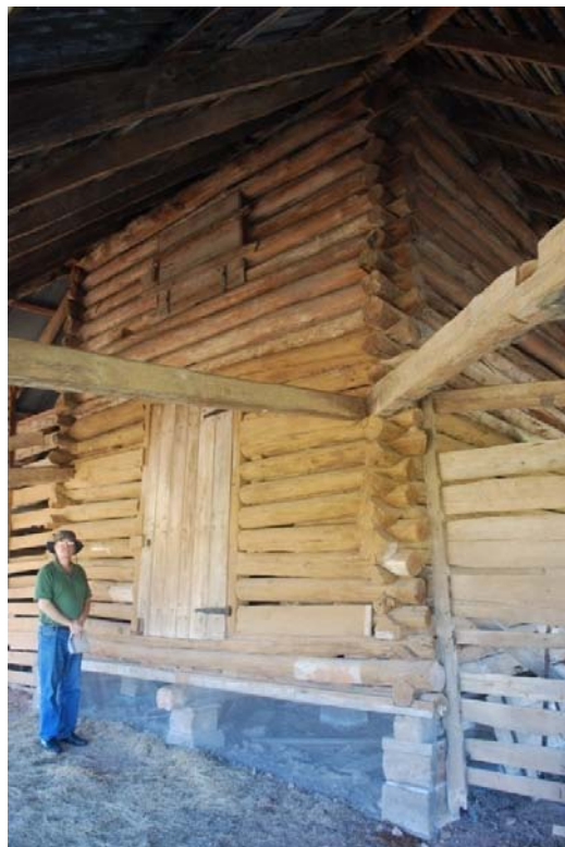
Photo 21. The unusual two story single crib of the Oakland barn.
