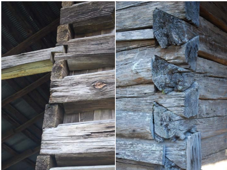
Photos 26 & 27. Square notch (left). Half dovetail notch (right).
