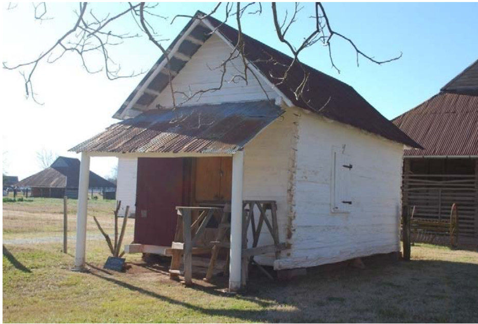
Photo 18. This single crib log building at Oakland Plantation, Natchitoches Parish is very finely crafted for a dependency (original use unknown). The whitewashing is relatively recent.
